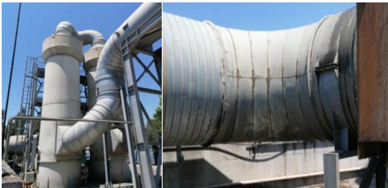
Figura 38 - Elementi in avaria: scrubber SCR 503 A/B, scrubber SCR 504
